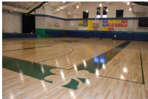
The Activity Center floor was resurfaced and painted this summer.
